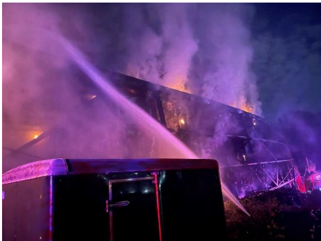
Railway Trestle Fire on August 20
