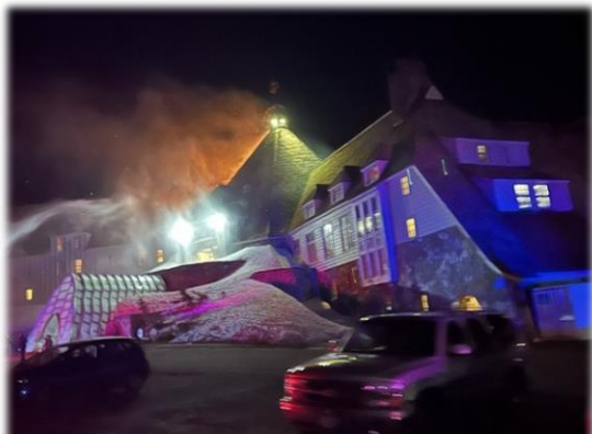
Timberline Lodge Fire
