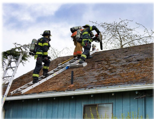
Destructive training on Silver Springs Road
