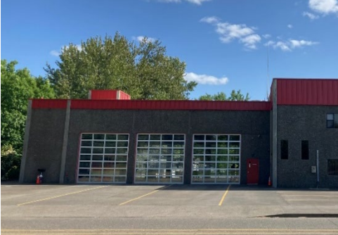
New bay doors at Station 1
